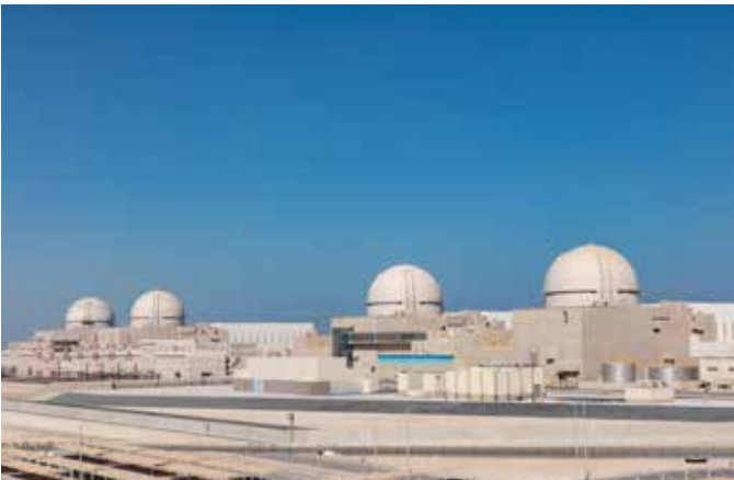
The Barakah Nuclear Energy Plant is currently delivering 4,200 MW megawatts of clean and reliable electricity to the UAE grid 24/7.
