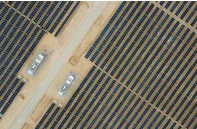
Mohammed bin Rashid Al Maktoum Solar Park in Dubai.
